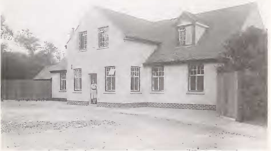
Fig. 16 Exterior of the British Mosquito Control Institute. Main entrance and driveway
